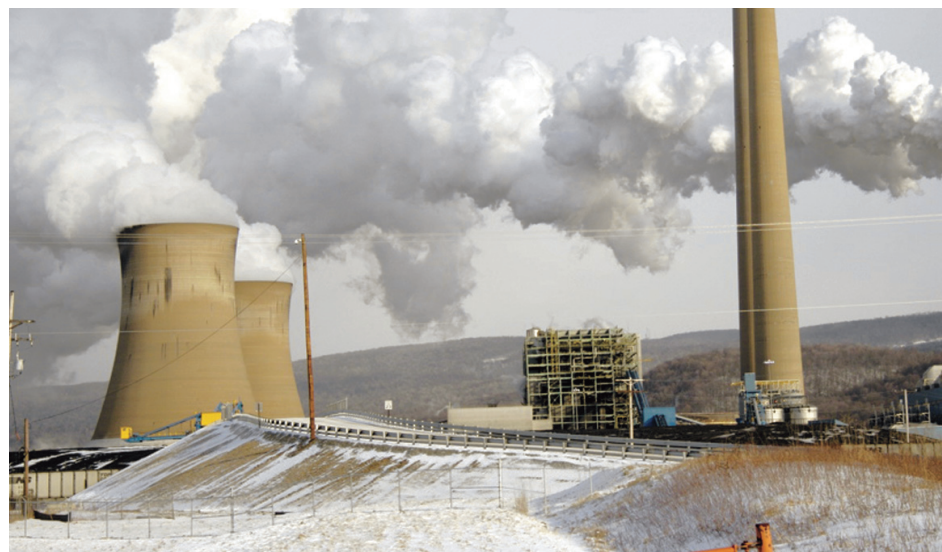
RRI Energy’s coal-fired power plant is situated on the Conemaugh River, west of Johnstown, PA.
