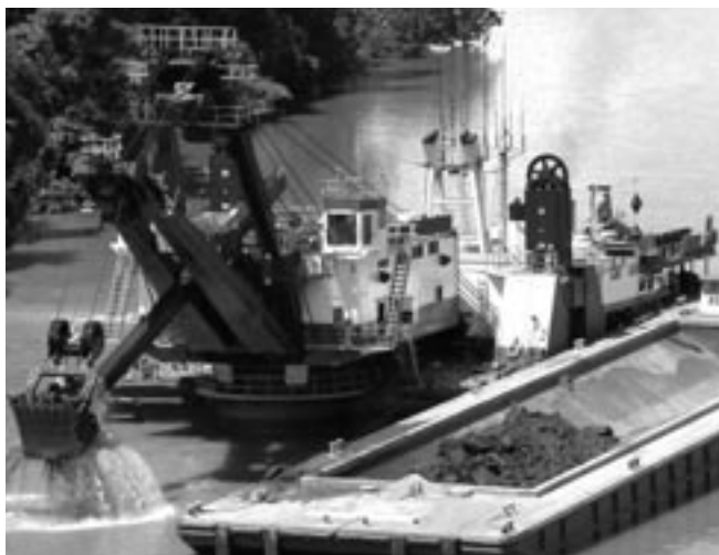
The Army Corps of Engineers proposes dredging dioxin-contaminated sediments from the Upper Saginaw River and disposing these sediments on a floodplain in Zilwaukee, Michigan. Above, a navigational river dredging operation.
